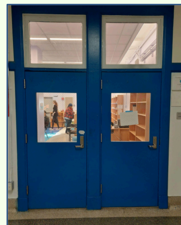
Doors to the 3rd Floor Library
